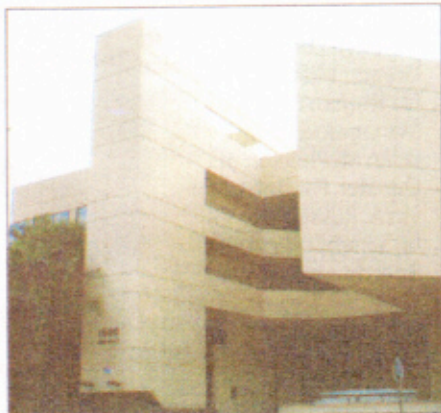
The Atrium at Coral Gables.
